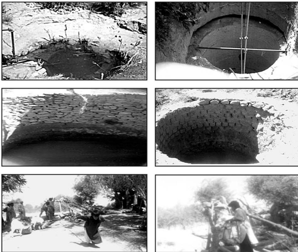
Figure 4. Different ways to draw water (dug wells, charkhi, small pumps)
